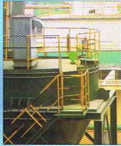
Sounding V at storage silo
